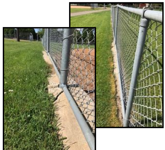
Examples of submerged or fractured concrete.
